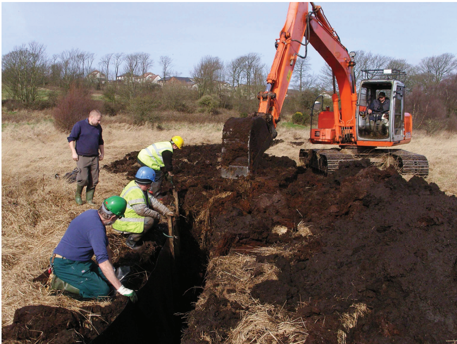
Installation of plygene sheeting at Heysham Moss.
